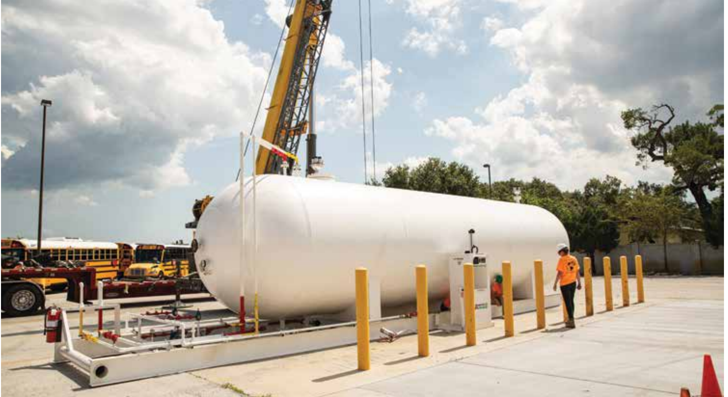
Above ground horizontal tank installation
