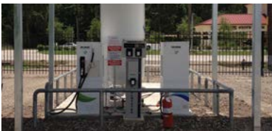
Above ground vertical tank installation
