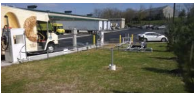
Below ground tank installation
