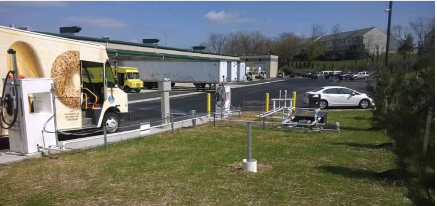
Below ground tank installation
