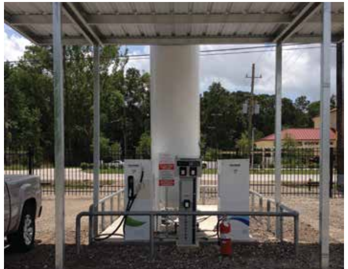
Above ground vertical tank installation
